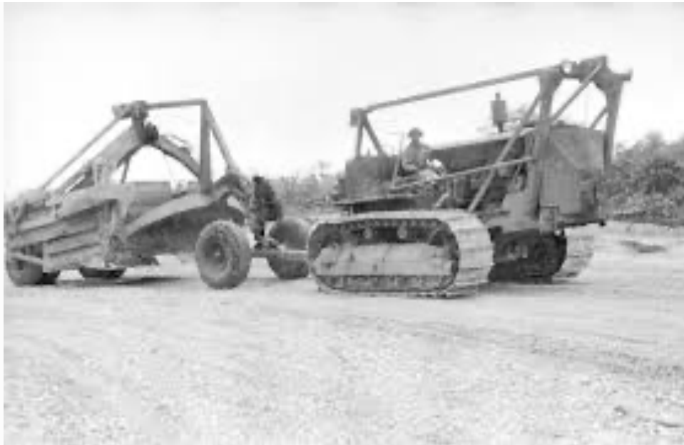
Sea Bee (CB) Construction Battalion Engineers constructing a critical jungle airfield
