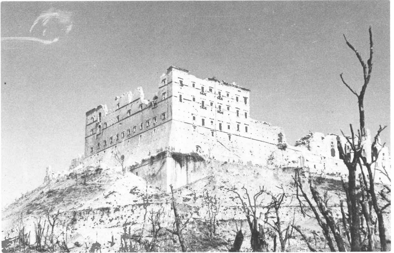
The ruins of the monastery after the fighting ended. While questions remain about the necessity of the abbey's bombing, there is little doubt about the damage done. Image: Polish National Digital Archives
