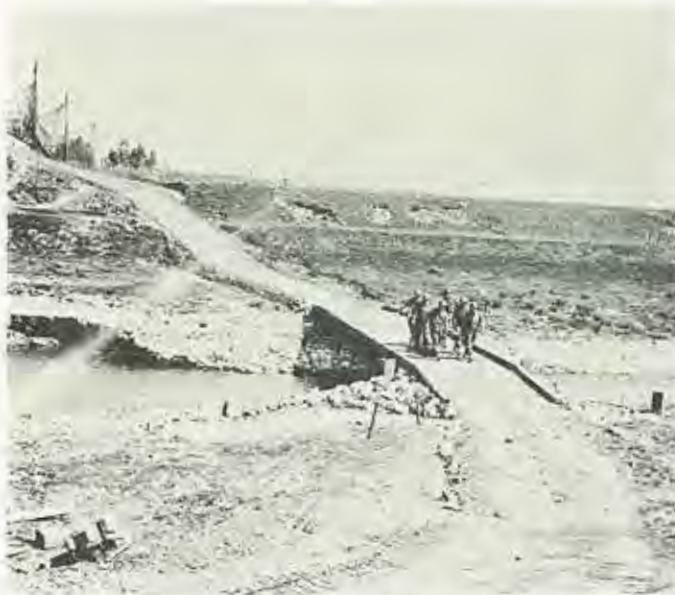
Members of the FSSF carrying logs across the Mussolini Canal to be used for bridgework and bunker fortifications. April 1944 (Durkee)
