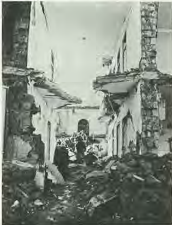
Forcemen moving into their barracks at Santa Maria (Capua-Vetere), demolished by the retreating Germans, 21 Nov 1943 Courtesy Maj. Gen. K.G. Wickham)
